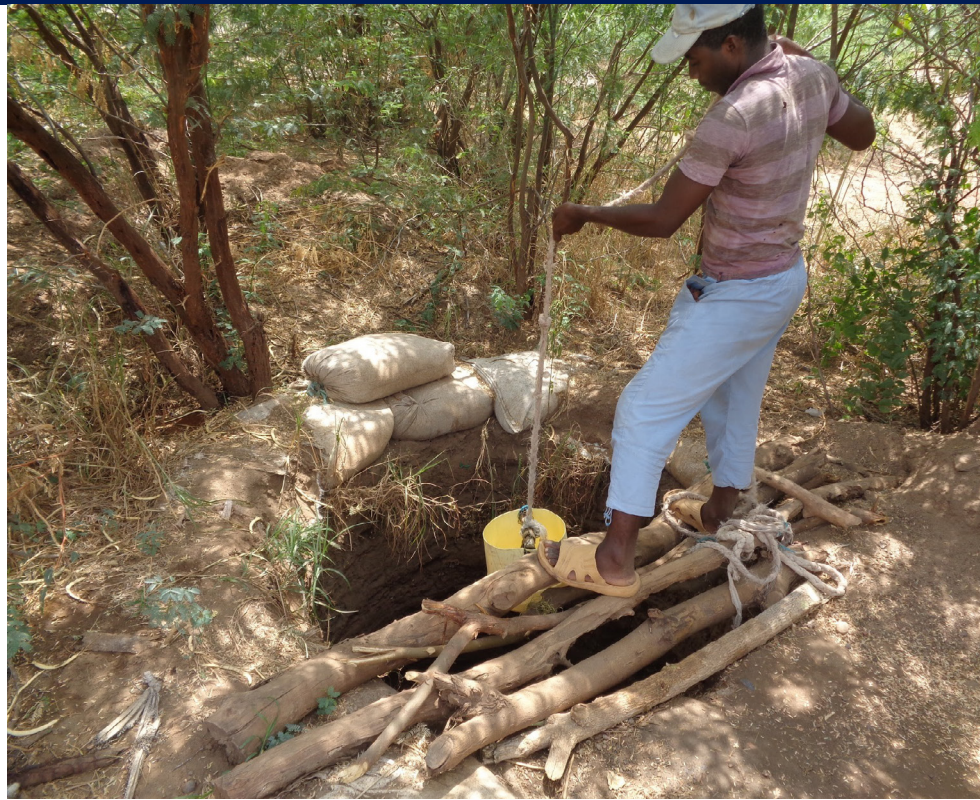
Well for groundwater, dug by refugees. Photo: Roland Kalamo
